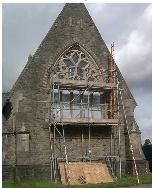
Glazing with polycarbonate in progress on the episcopal Chapel
