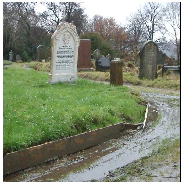
Damaged timber edging near grave of Balloon Girl
