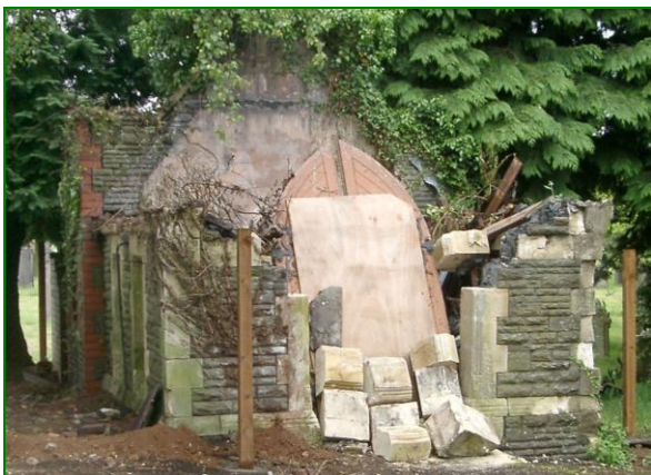
Collapsed Bier House Wall
