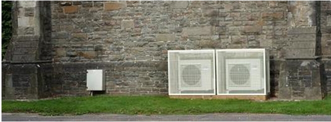
Air-conditioning unit at front of Non-conformist Chapel
