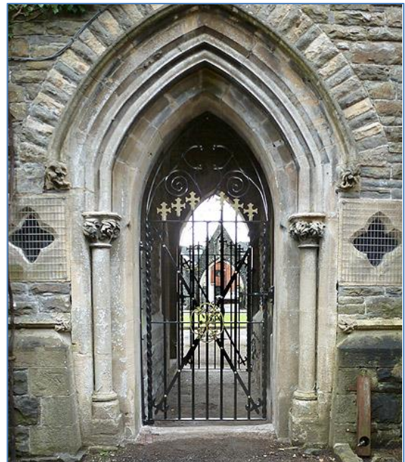
The gated central passage
