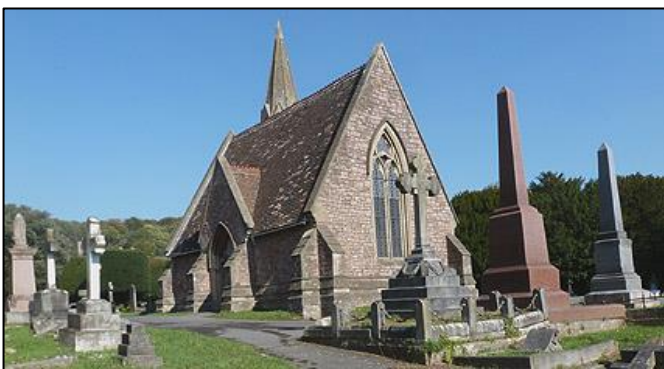
Restored Anglican Chapel
