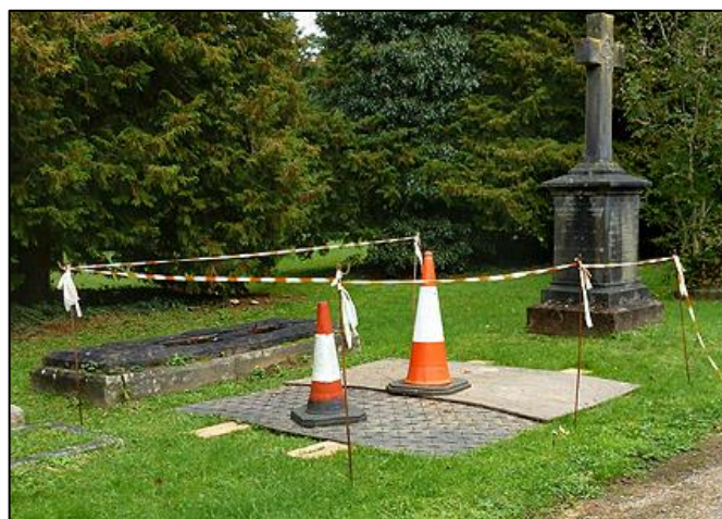
Collapsed vault in Section C plated over for safety
