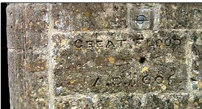
Flood mark on St Thomas' Church, Redwick
