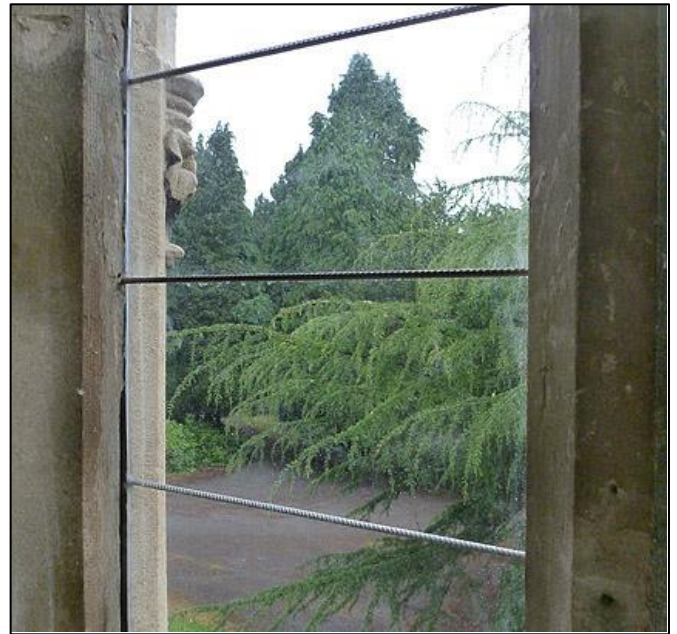
View from first floor of bell tower
