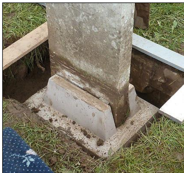
CWGC headstone mounted in saddle, before backfilling the hole
